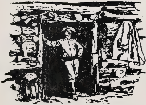
D. B. Healey's livery stable, erected at Beaver City in spring 1886. Three walls were dirt banks, and front of logs.
